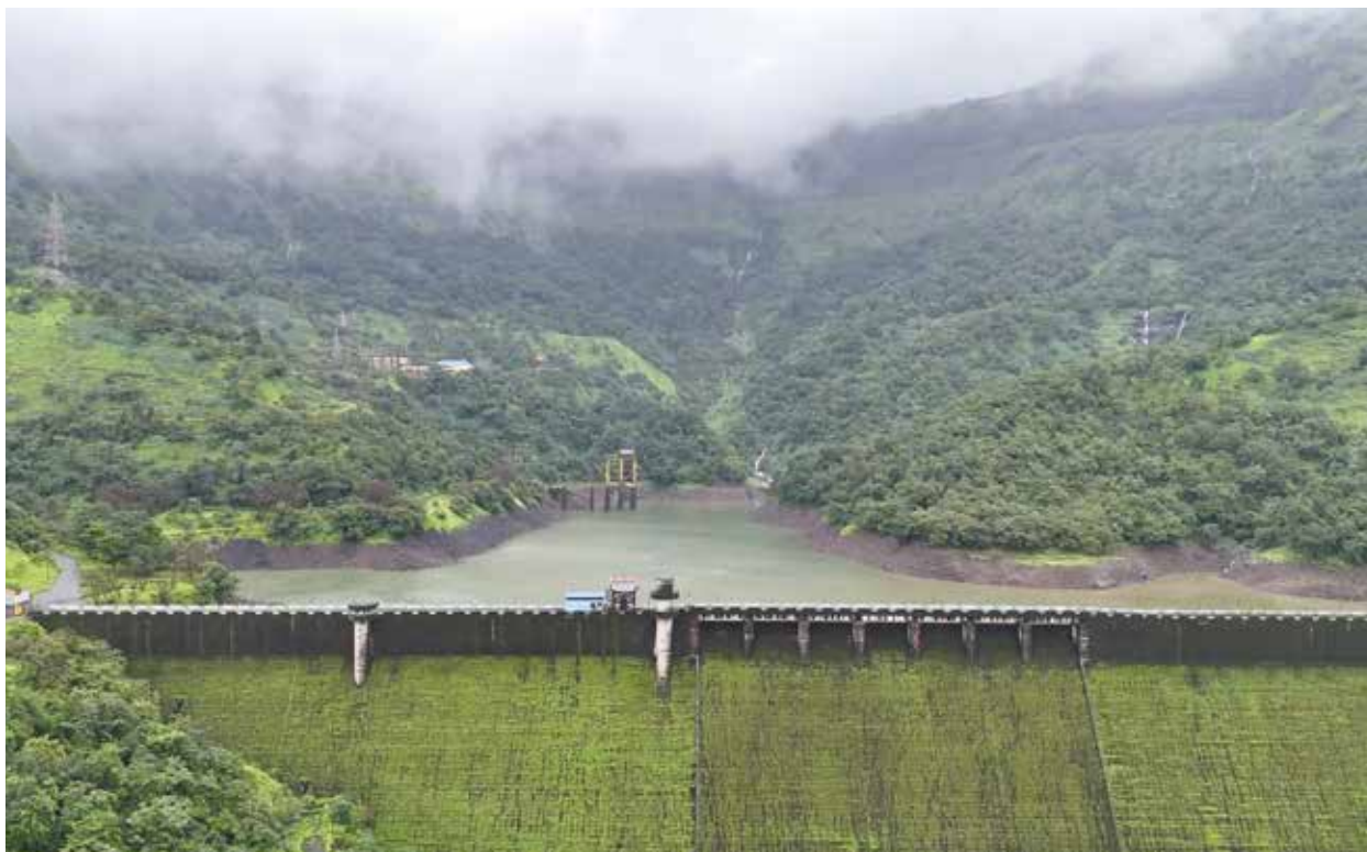
HPS Ghatghar Dam
