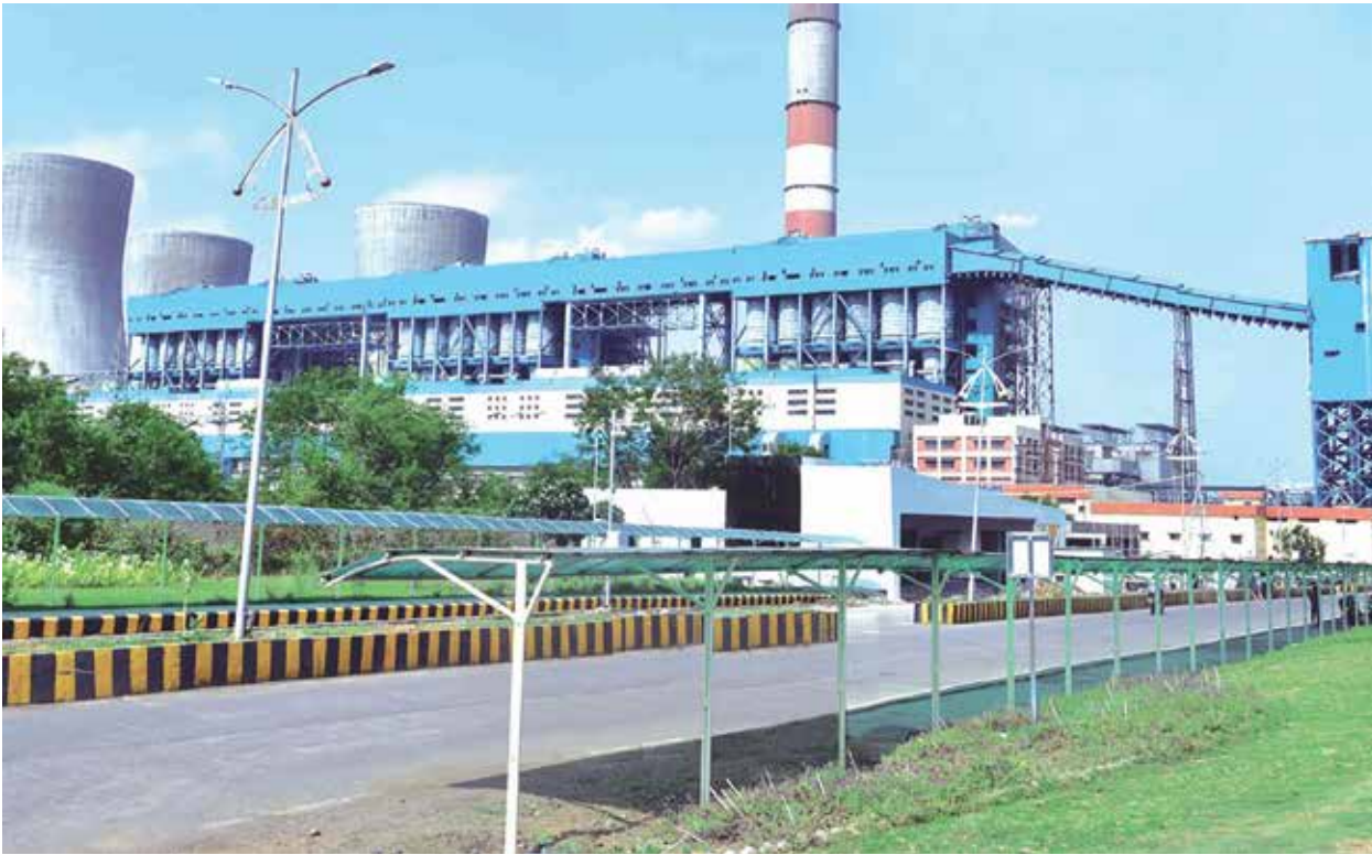
Koradi Thermal Power Station
